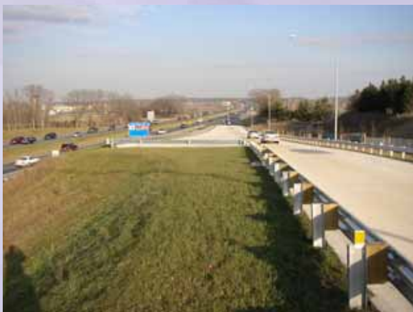
I-70 roadway that was awarded the 2004 Excellence in Concrete Award from the American Concrete Institute.
